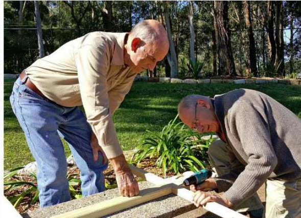
Ross and Hetta assembling the roof frame
